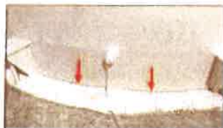
Minor separation of water proofing membrane at tank shell
